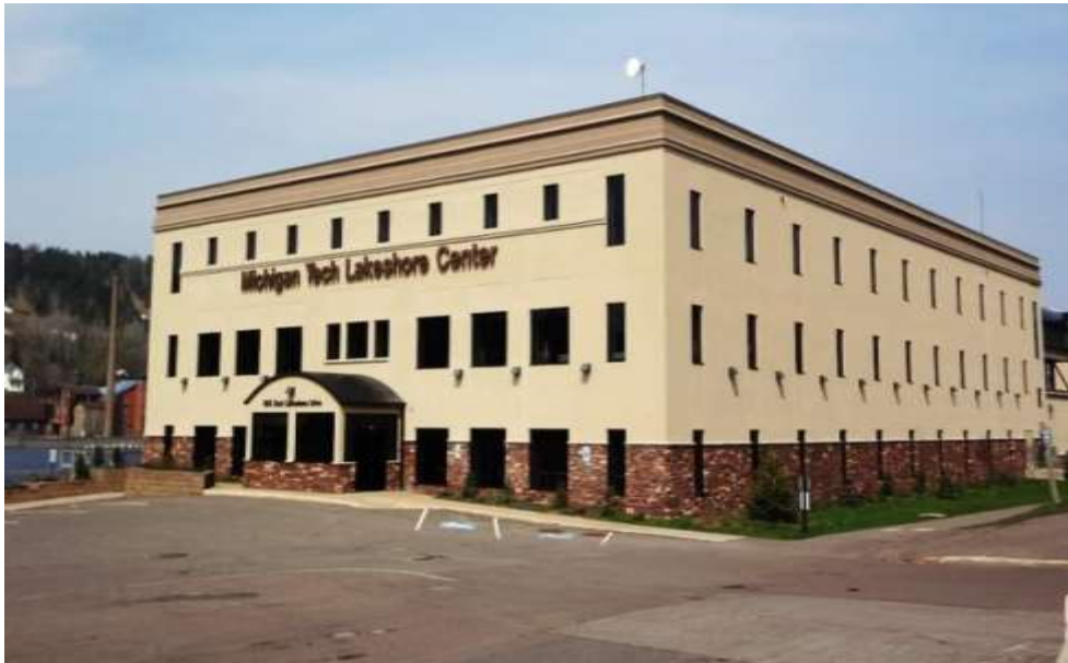
Figure 2.4: Test Bed – Lakeshore Centre, Michigan Technological University [See Appendix C for documentation of permission to republish this material]
